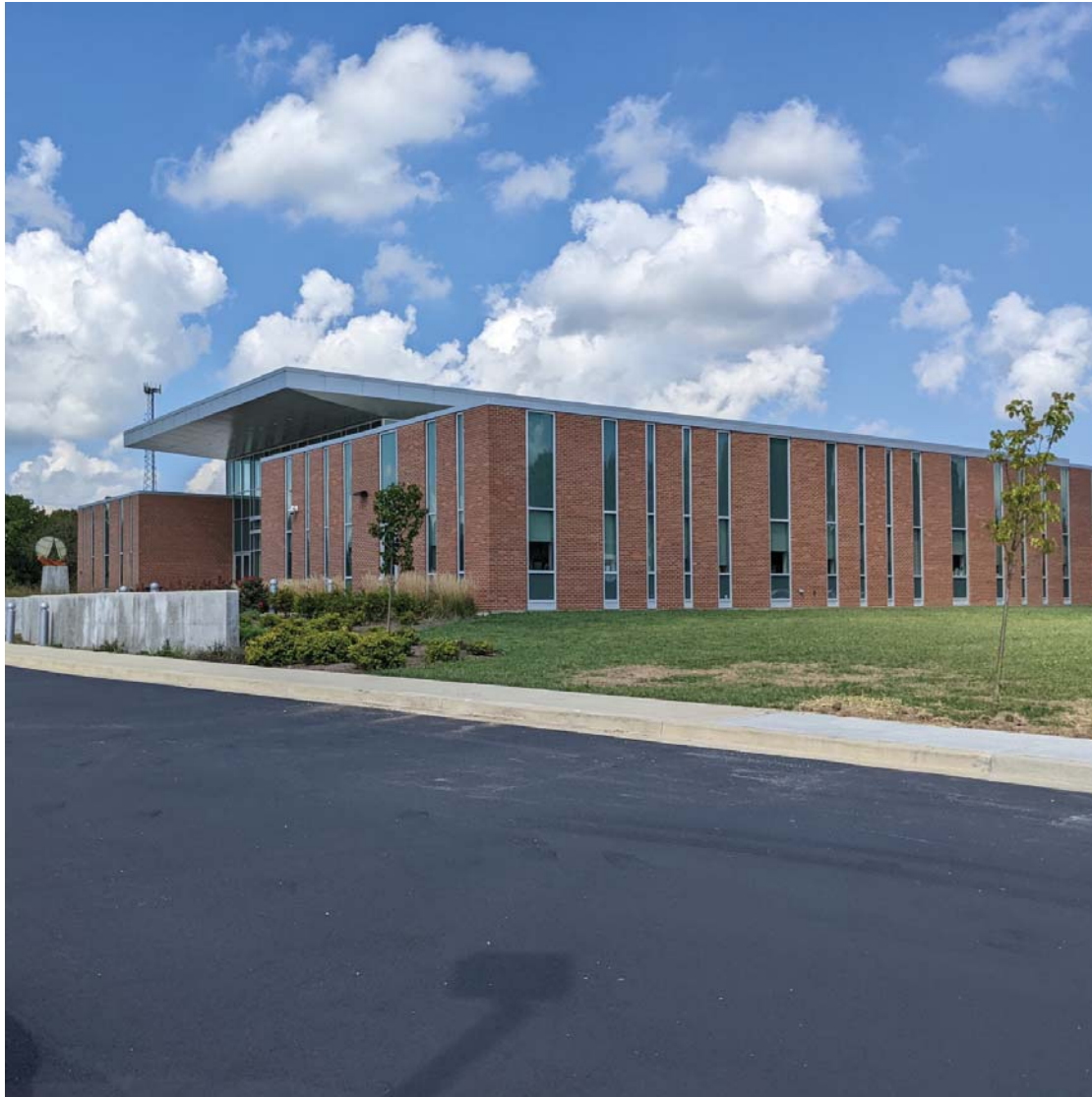
BLDG NO. LL02
